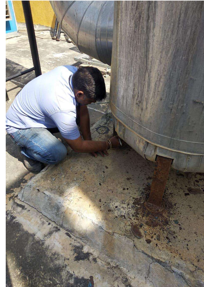
Expansion Tank Cleaning – 2 AB
