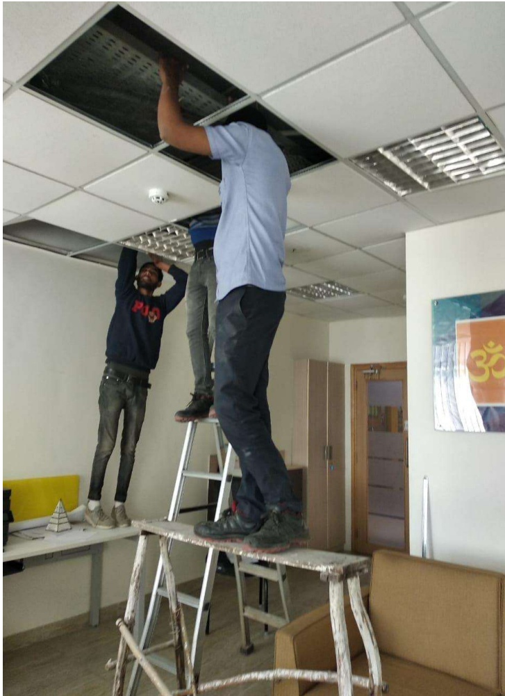
AC Unit installation in Purchase Office
